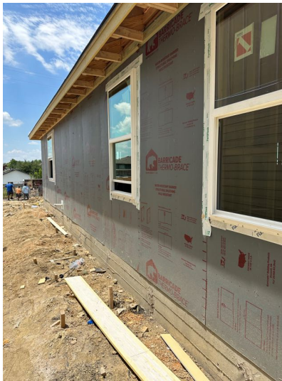
INSTALL PARGE COAT
