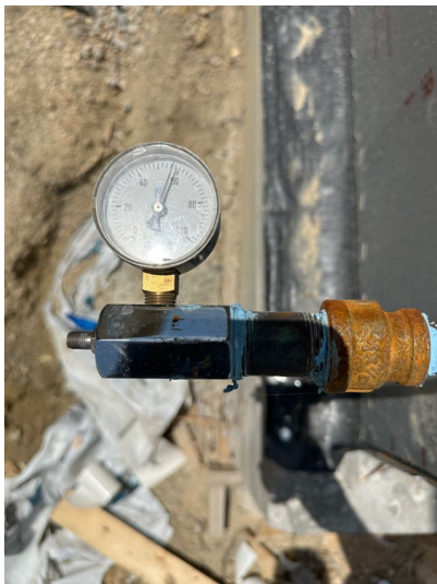
PRESSURE TEST UNDERWAY
