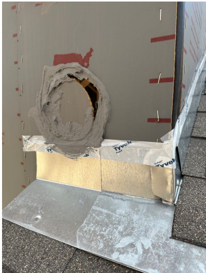
SEAL HOLES COMPLETELY
