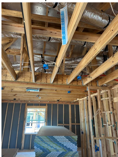
JOIST HANGERS IN PLACE
