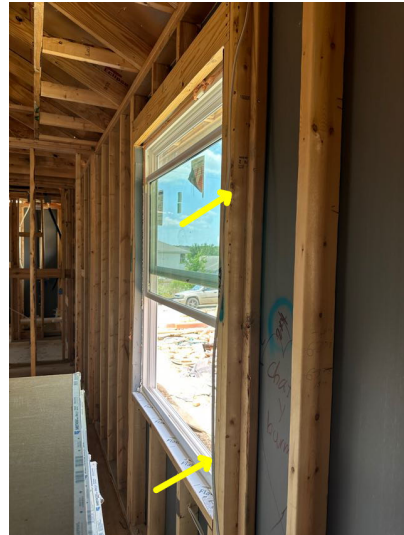
SECURE LOOSE WIRE
