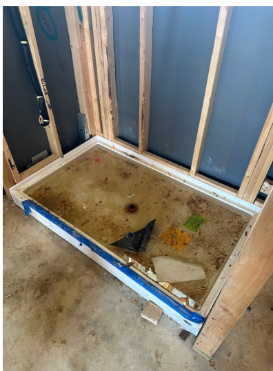
LEAK TEST UNDERWAY
