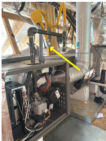
GAS LINE PREPPED
