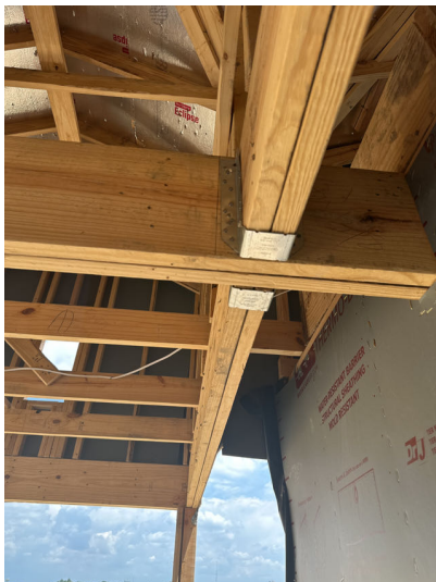
JOIST HANGERS IN PLACE
