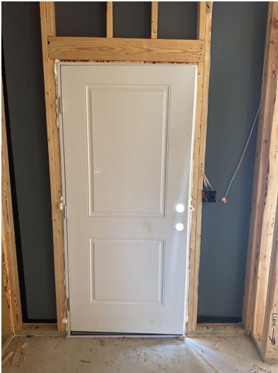
FRONT DOOR INSTALLED
