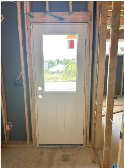
BACK DOOR INSTALLED
