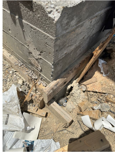
FORM BOARDS LEFT IN PLACE
