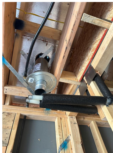
VENT AND PLUMBING SUPPLY PREPARED
