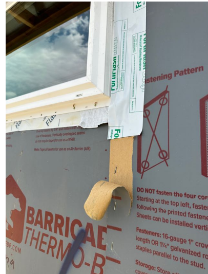
REPAIR MOISTURE BARRIER
