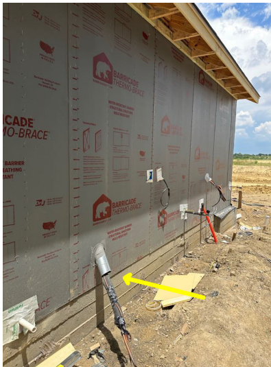
CONDENSER LOCATION PREPPED
