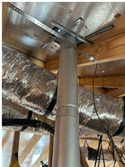
PROPER VENT CLEARANCE
