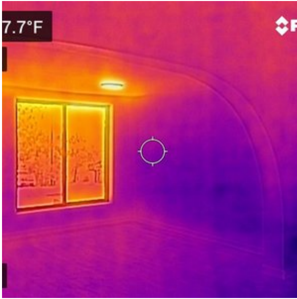
THERMAL CAMERA: NORMAL READINGS
