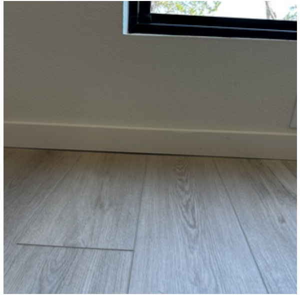
AREAS OF UNEVEN FLOOR SURFACES
