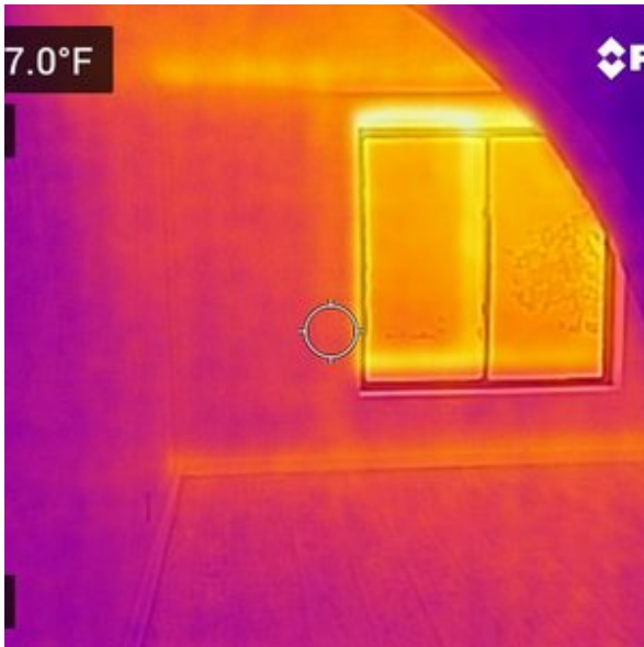
THERMAL CAMERA: NORMAL READINGS
