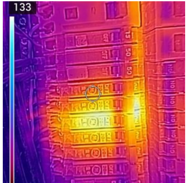
THERMAL CAMERA: NORMAL READINGS
