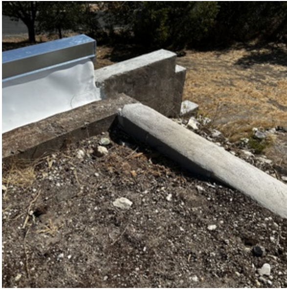
PREVIOUS ROOF/WALL REPAIRS
