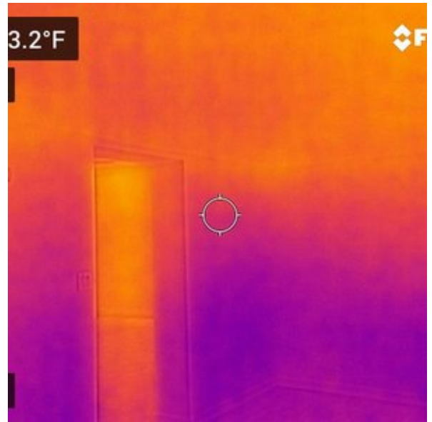
THERMAL CAMERA: NORMAL READINGS
