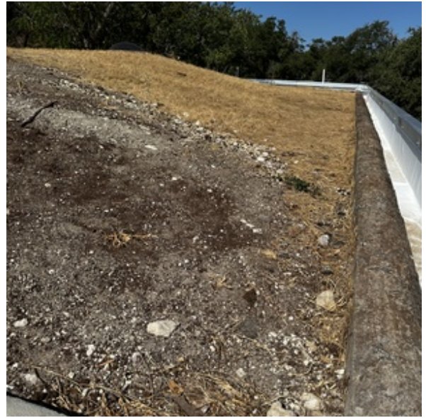
FRONT ROOF GUTTER PROVIDED
