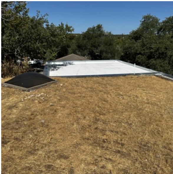
UNIQUE DRAINAGE NEEDS AT ROOF
