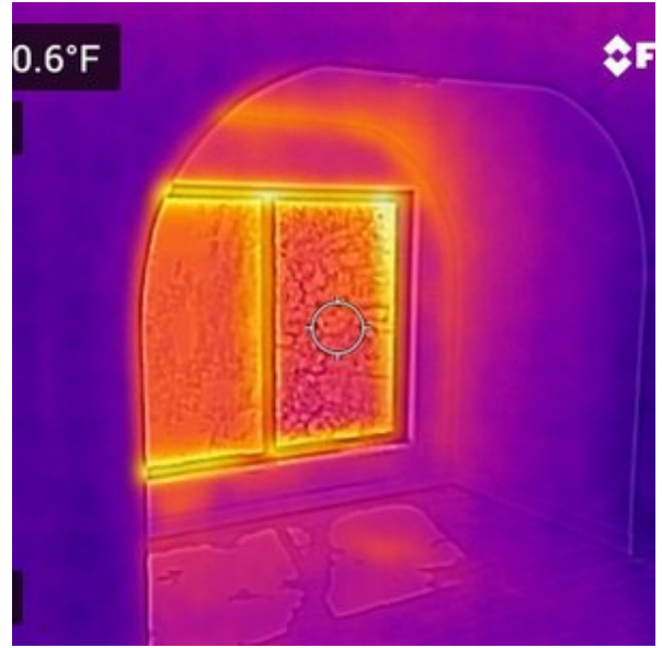
THERMAL CAMERA: NORMAL READINGS
