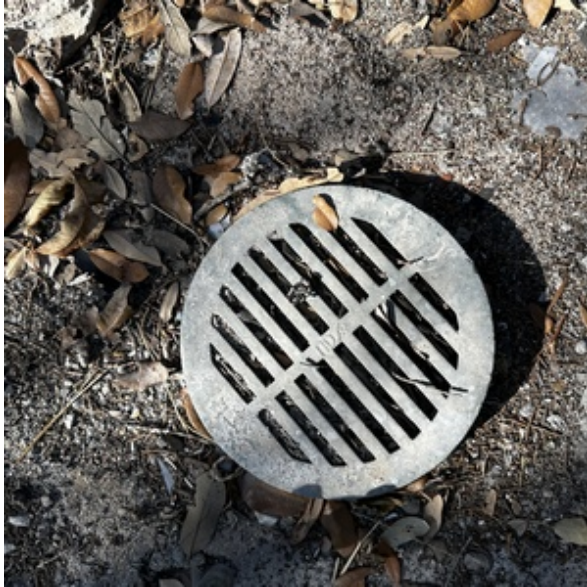
SUB-GRADE DRAINS PRESENT
