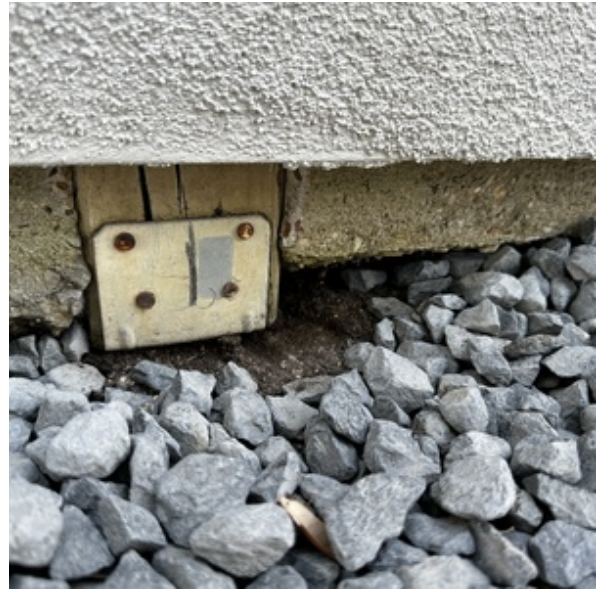
4X4" POST AT GARAGE SLAB
