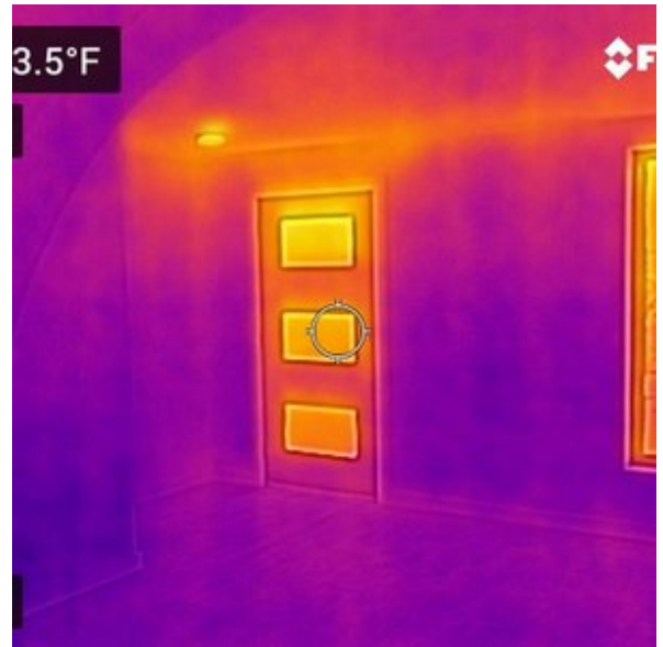
THERMAL CAMERA: NORMAL READINGS
