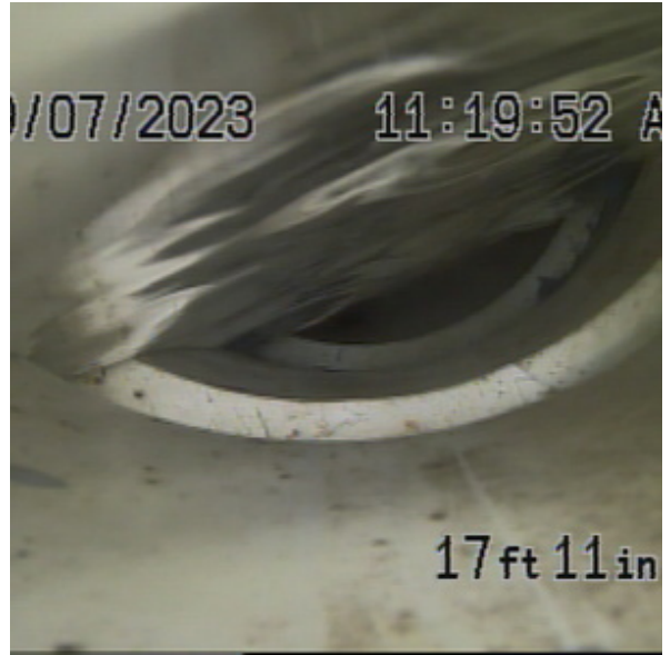
NORMAL DRAINAGE OBSERVED
