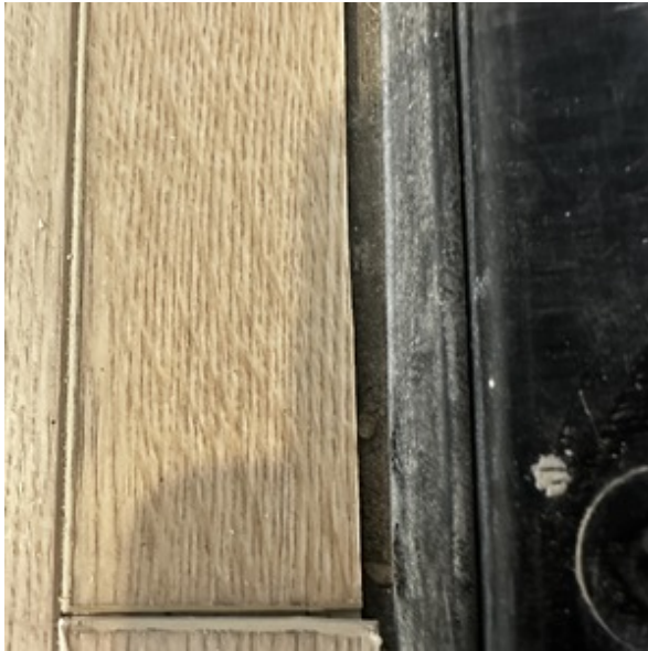
SEAL GAPS AT TRANSITIONS
