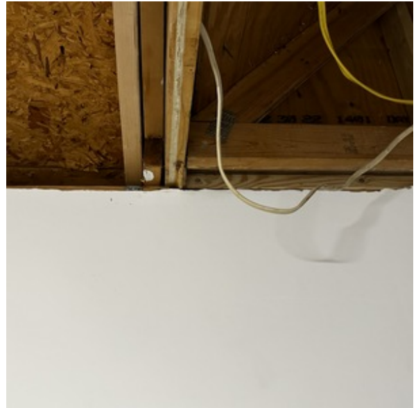
UNSECURED WIRING
