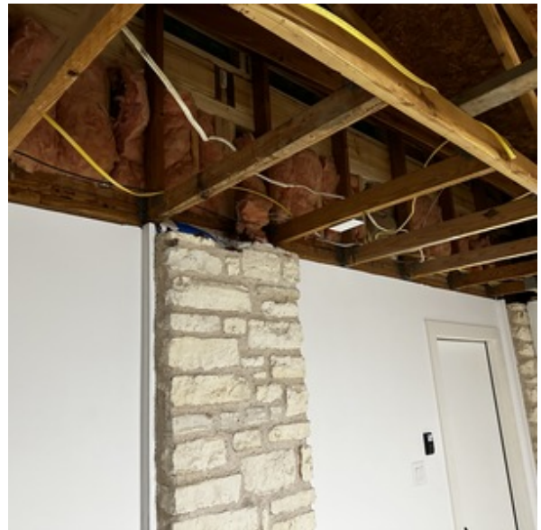
ENGINEERED TRUSS AT GARAGE
