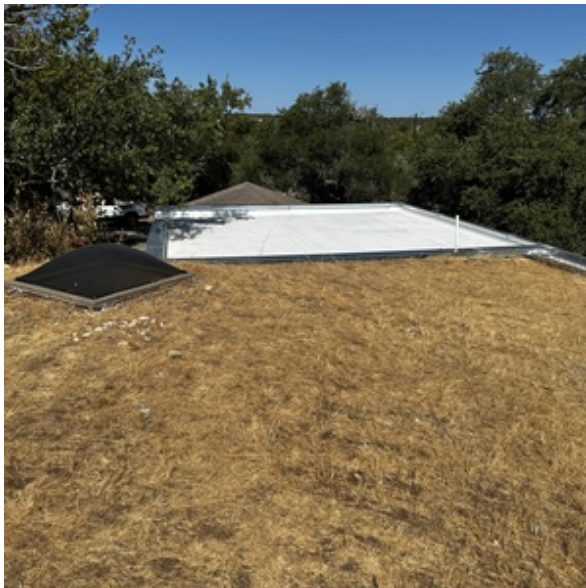
MULTIPLE ROOF COVERING TYPES
