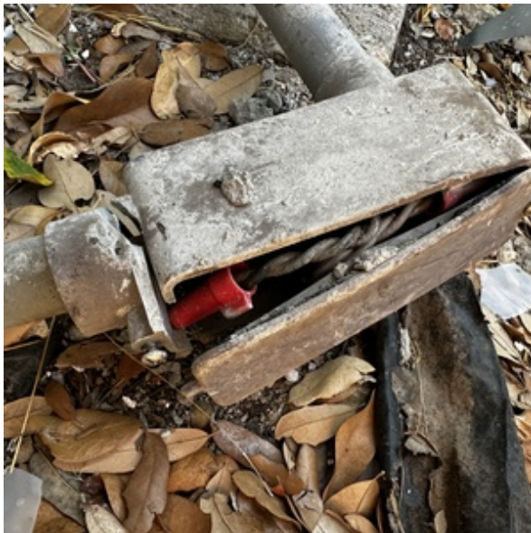
OPEN/DAMAGED J-BOXES
