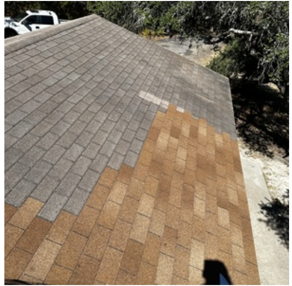
PARTIAL SHINGLE REPLACEMENT
