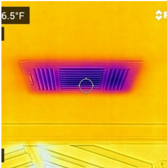
THERMAL CAMERA - NORMAL READINGS
