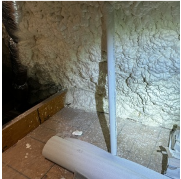
FOAM APPEARS TO MEET STANDARDS
