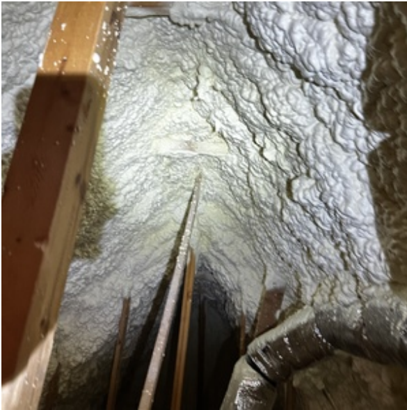
FRAMING SUPPORTS PRESENT
