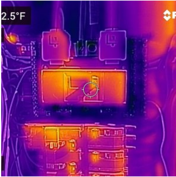
THERMAL CAMERA - NORMAL READINGS
