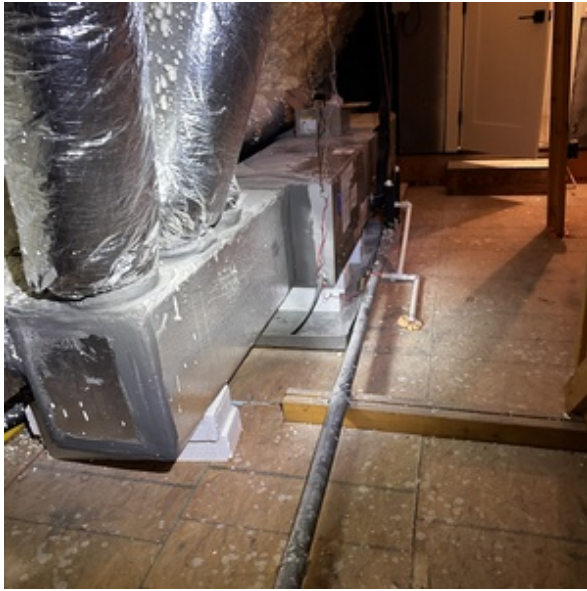
INSTALL MEETS STANDARDS
