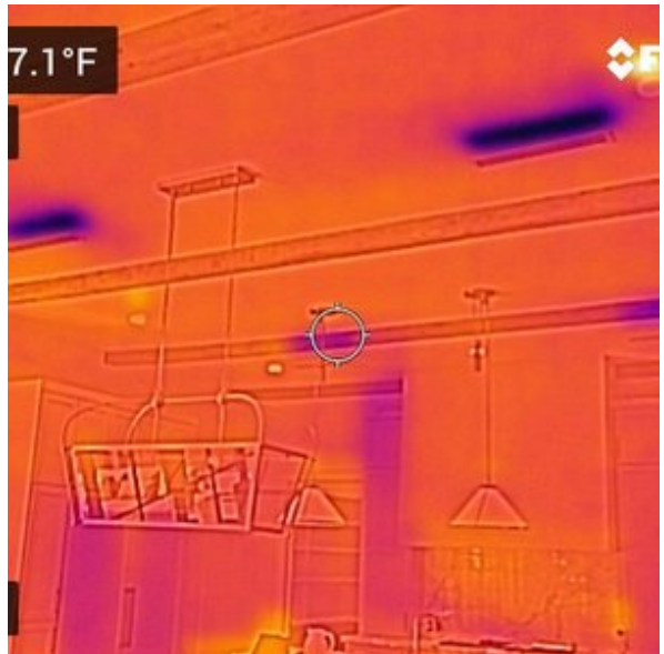
THERMAL CAMERA - NORMAL READINGS
