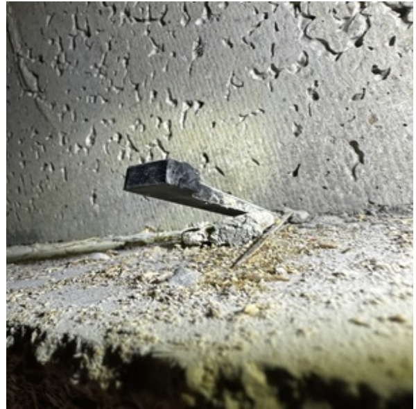
CUT/REMOVE PLASTIC SHIM
