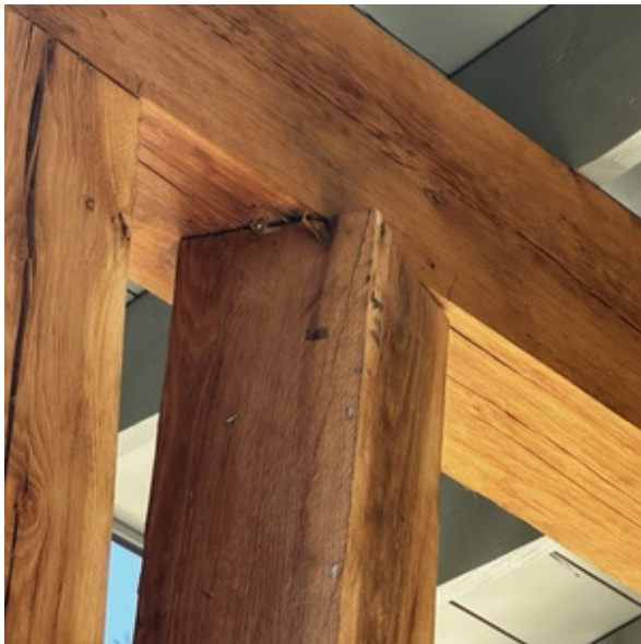
BOWED/TWISTED COLUMN
