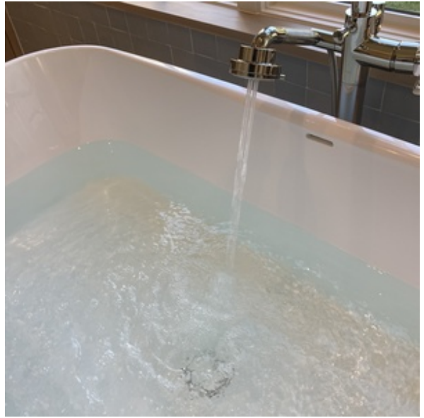
DRAIN/LEAK TESTING CONDUCTED
