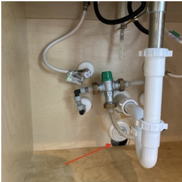
DRAIN/LEAK TESTING CONDUCTED
