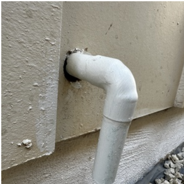
CAULK/SEAL AT PENETRATIONS
