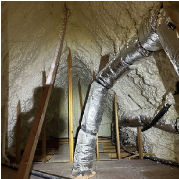
BACK ATTIC SPACE
