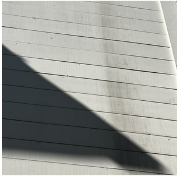
AREA OF ROOF RUN-OFF
