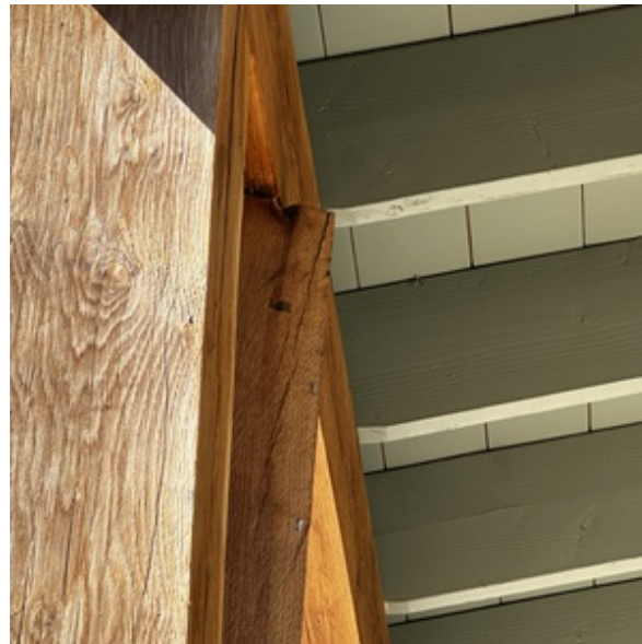
BOWED/TWISTED COLUMN
