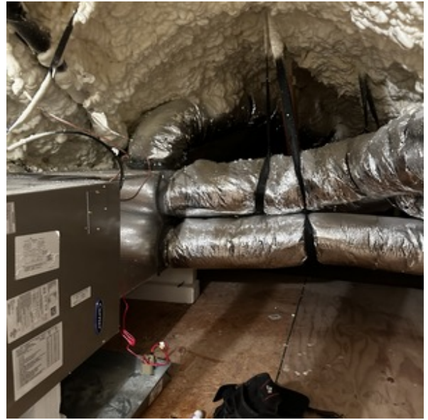
2ND FLOOR UPPER ATTIC
