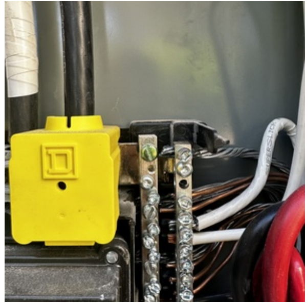
PROPER PANEL BONDING
