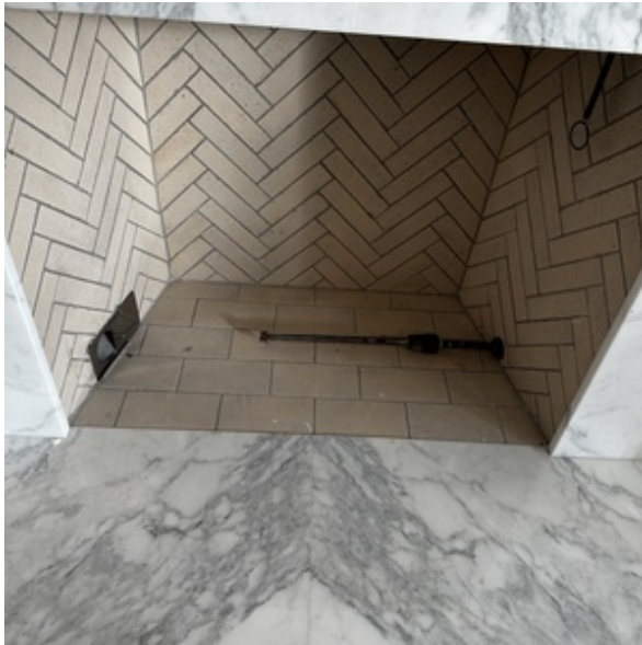
FIREWALL IN GOOD CONDITION
