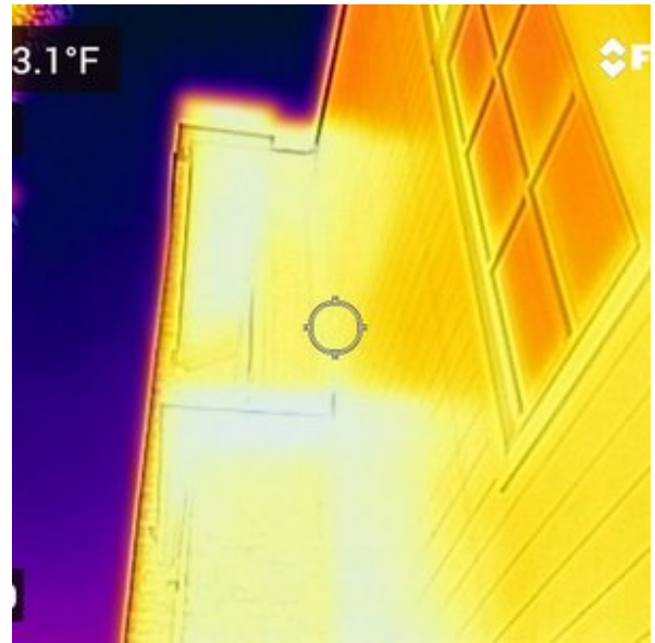
THERMAL CAMERA - NORMAL READINGS
