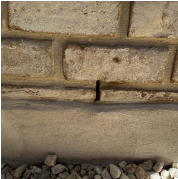
WEEP HOLES PROVIDED IN MOST AREAS
