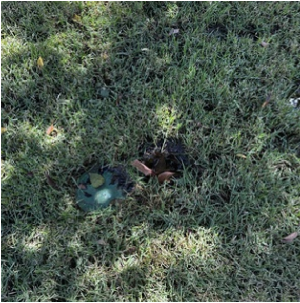
DRAIN TERMINATION NEAR STREET
