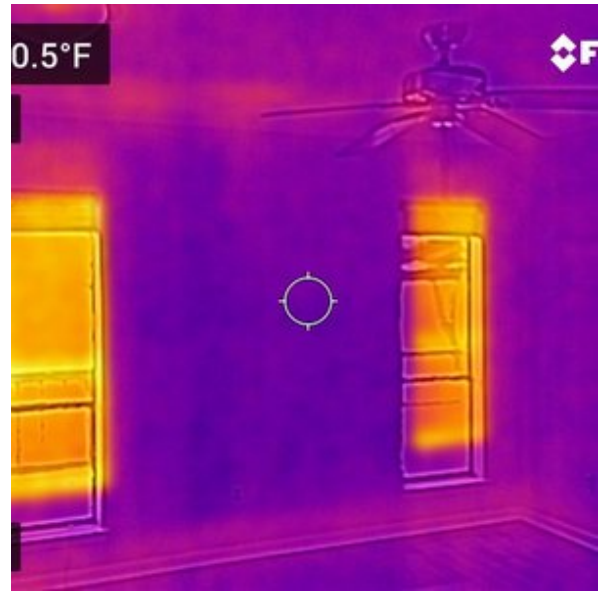
THERMAL CAMERA - NORMAL READINGS
