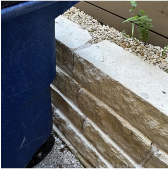
RETAINING WALL PROVIDED
