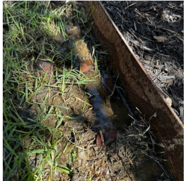
FRONT YARD: SOIL SATURATION
