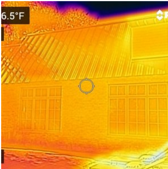
THERMAL CAMERA - NORMAL READINGS
