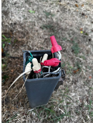
ELECTRICAL SERVICE NEEDS
