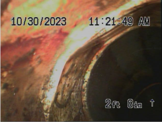
ATTEMPTED ENTRY TOWARDS BUILDING AT MAIN CLEAN OUT
