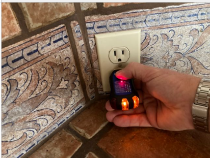
GFCI UPDATE NEEDS
