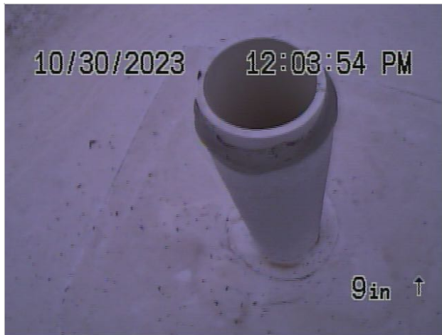
ENTRY FROM ROOF LEVEL (V1)
