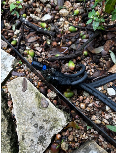
ELECTRICAL SERVICE NEEDS
