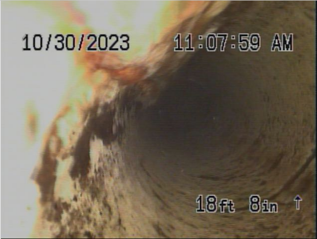
PROPER DRAINAGE TO OSSF
