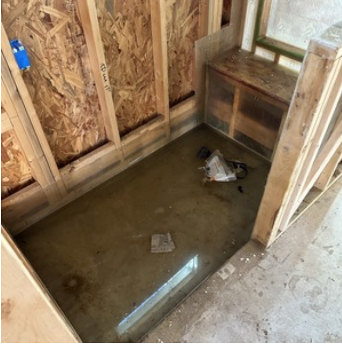
PLUMBING TESTS UNDERWAY
