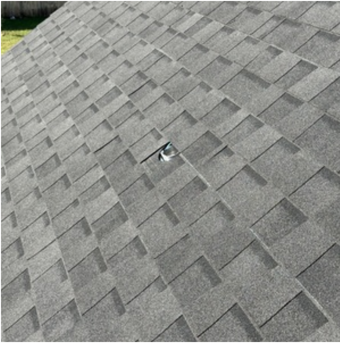
FULLY DRY IN PRIOR TO DRYWALL
