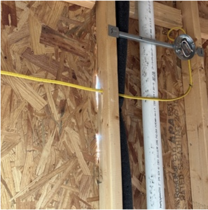
SEAL GAPS AS NEEDED
