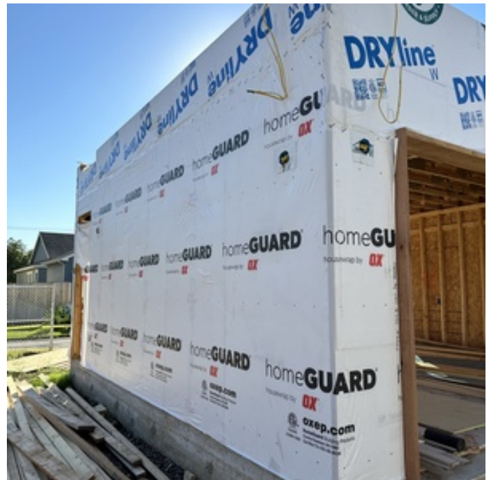
ENSURE INCOMPLETE CIRCUITS FINISHED
