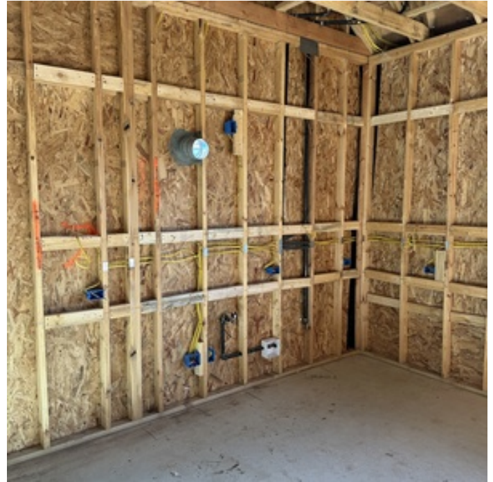
PROPER PLATING OBSERVED
