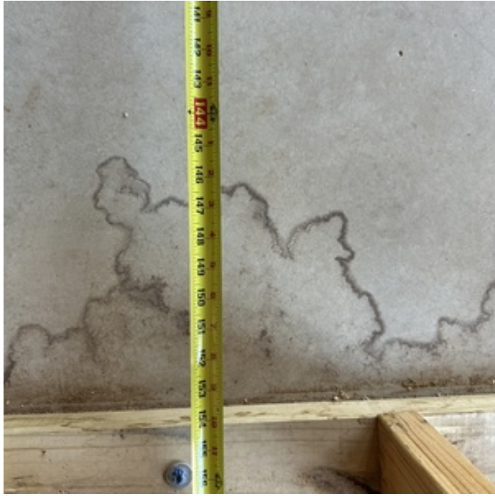
ENSURE ALL FRAMING DRY PRIOR TO INSTALLS
