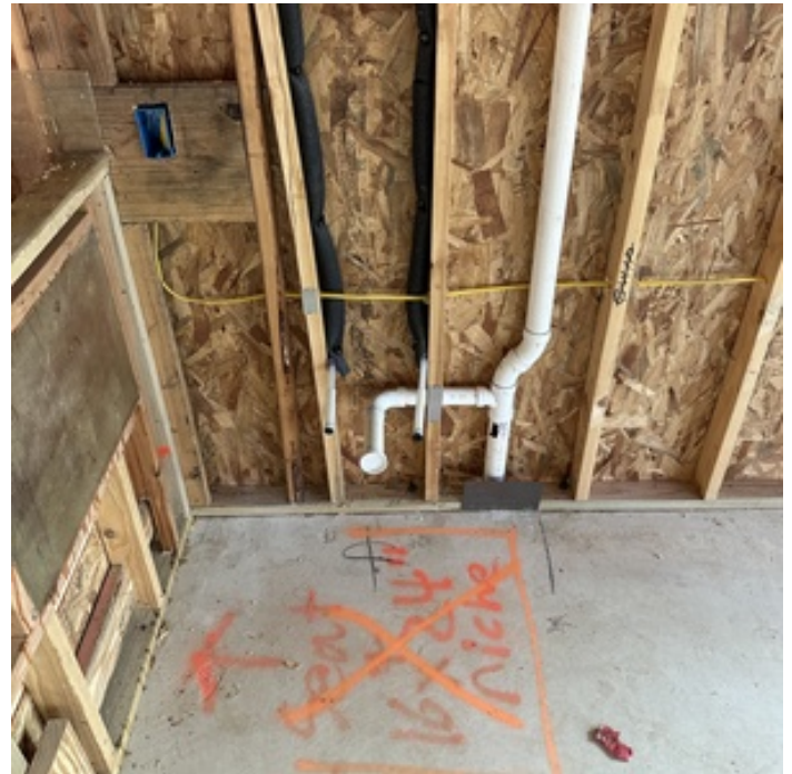
PROPER PLUMBING PLATING
