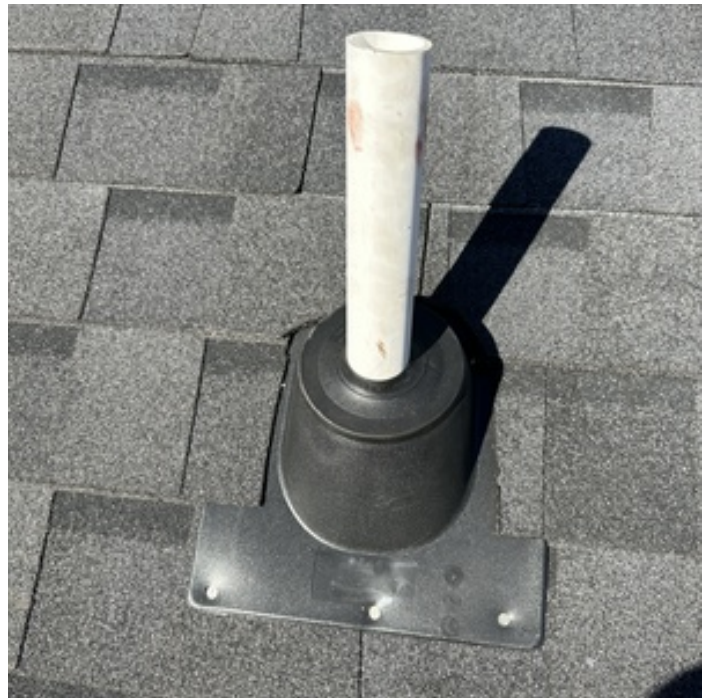
SEAL NAILS, PAINT PROTECT PVC
