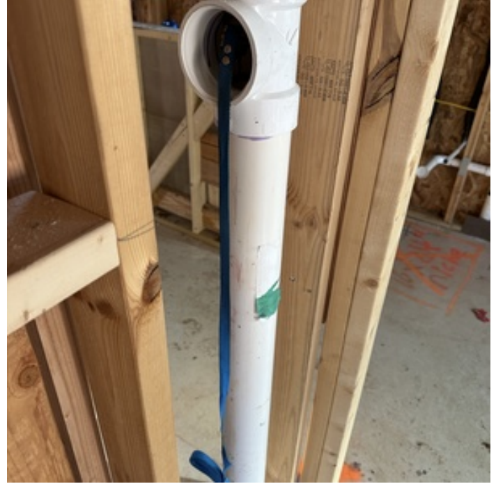
LEAK TESTING UNDERWAY
