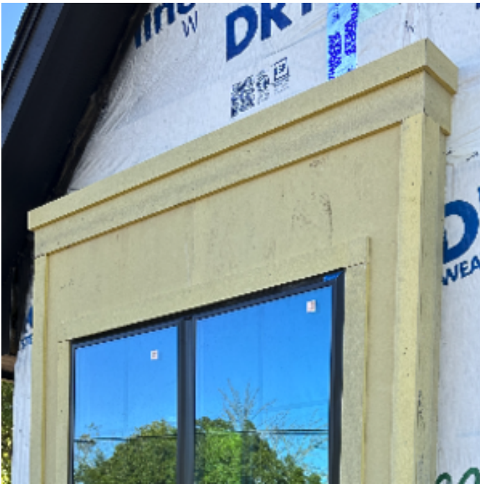
ENSURE PROPER FLASHING/PROTECTION
