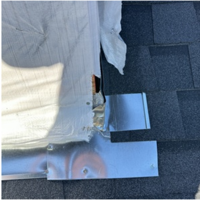
ADDRESS MINOR BARRIER FLAWS
