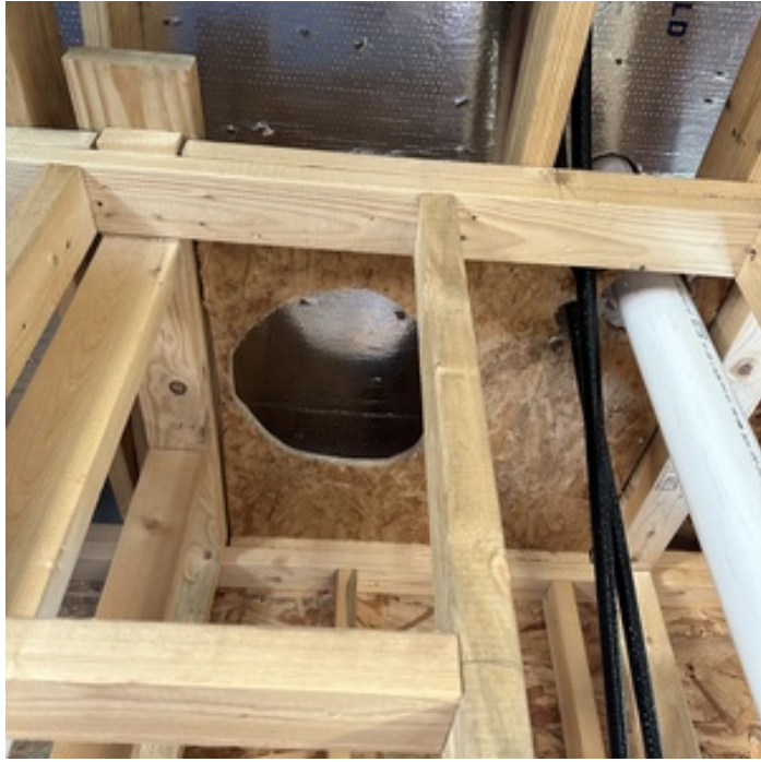
FIRE SEAL AS NEEDED
