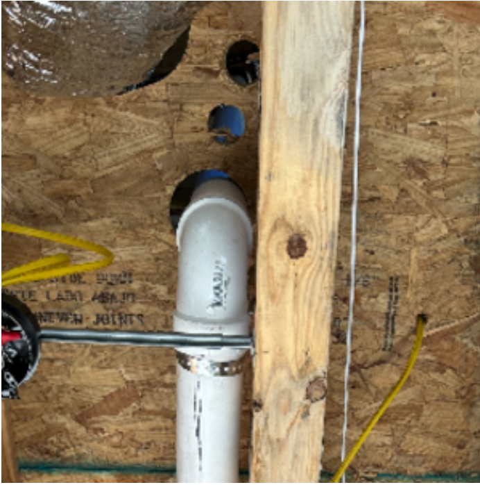
SEAL ALL BOREHOLES
