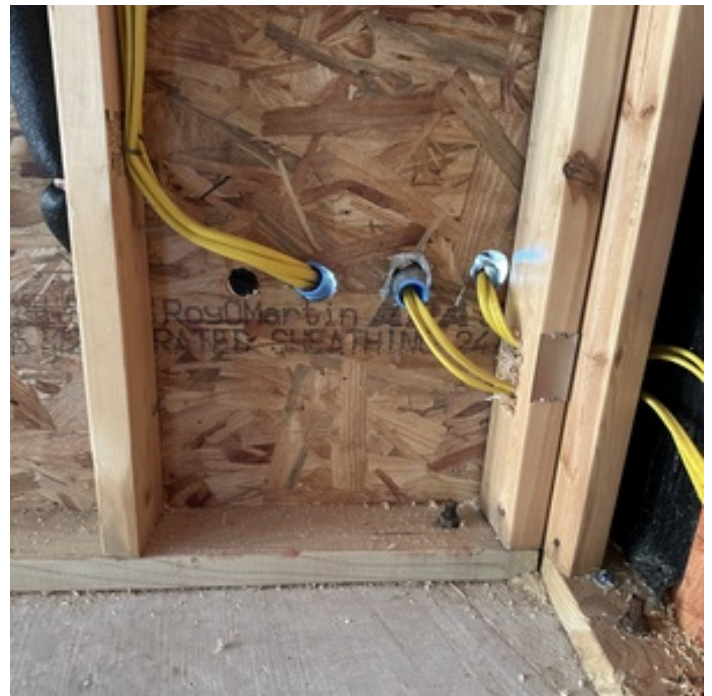
SEAL GAPS AS NEEDED
