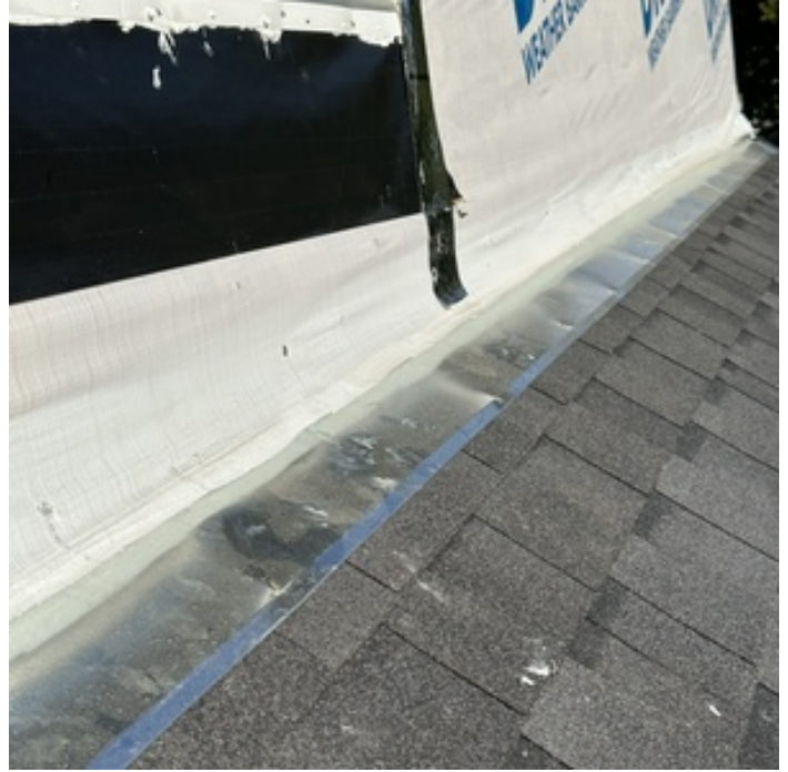
PROPER FLASHING INSTALL
