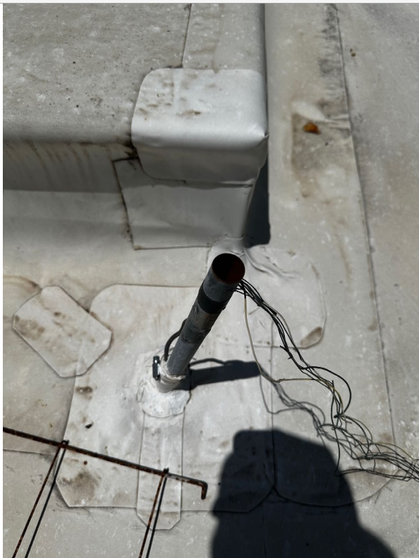
ROOF LEAK POINTS
