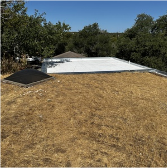
MULTIPLE ROOF COVERING TYPES
