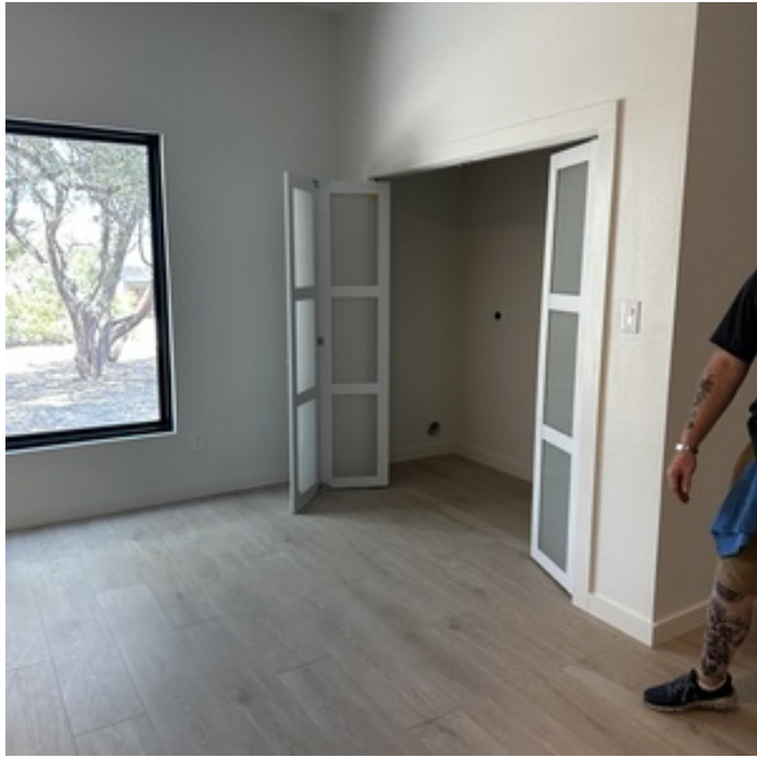
LEAK DISCOVERED IN LAUNDRY
