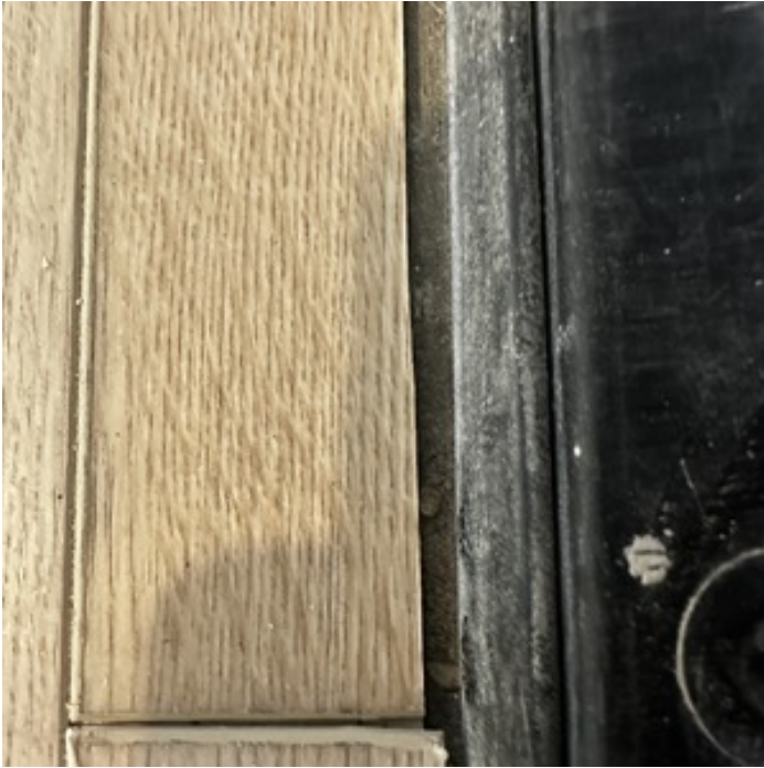
SEAL GAPS AT TRANSITIONS
