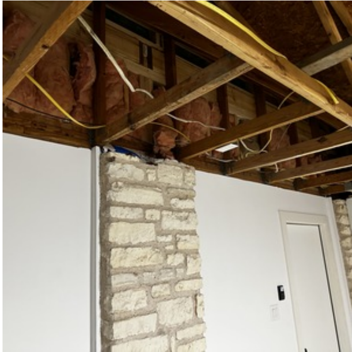
ENGINEERED TRUSS AT GARAGE
