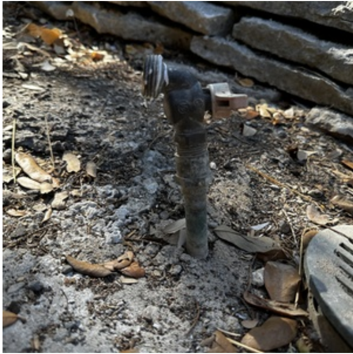
PROTECT PIPE, ADD ANTI-SIPHON
