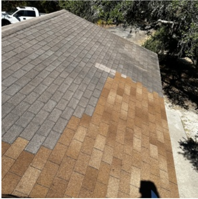
PARTIAL SHINGLE REPLACEMENT
