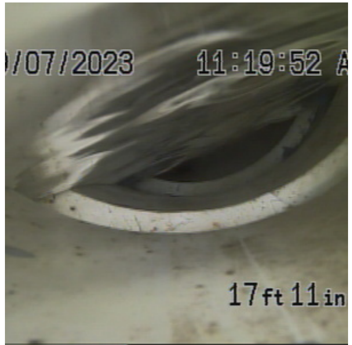
NORMAL DRAINAGE OBSERVED
