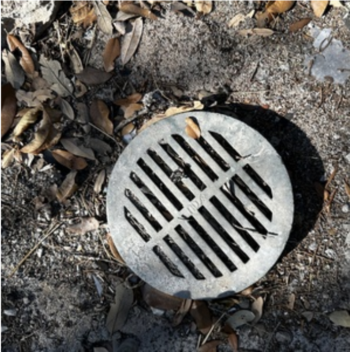
SUB-GRADE DRAINS PRESENT
