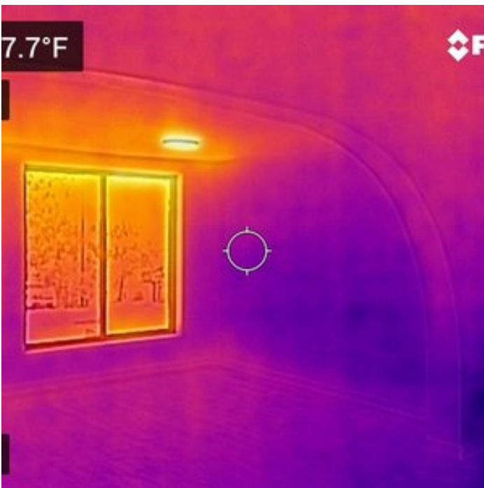
THERMAL CAMERA: NORMAL READINGS
