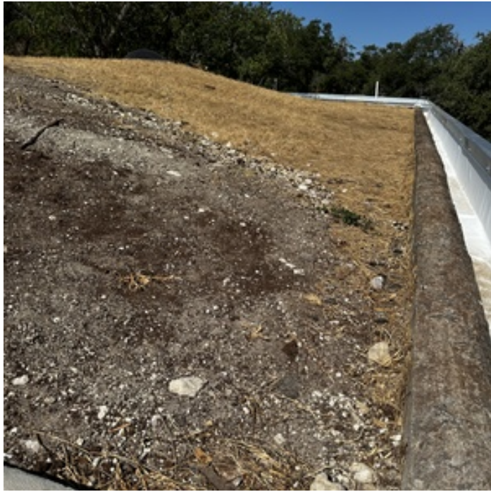
FRONT ROOF GUTTER PROVIDED
