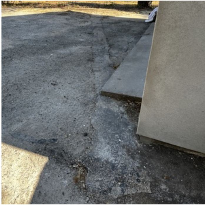
CUT/PATCH: PREVIOUS PIPE REPAIR
