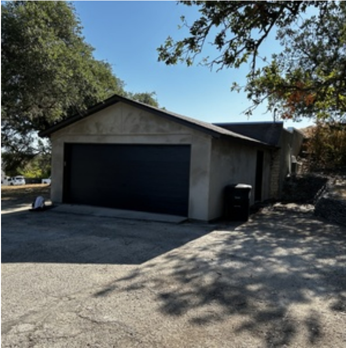
TYPICAL DRIVEWAY FLAWS
