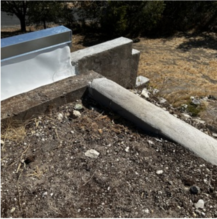
PREVIOUS ROOF/WALL REPAIRS
