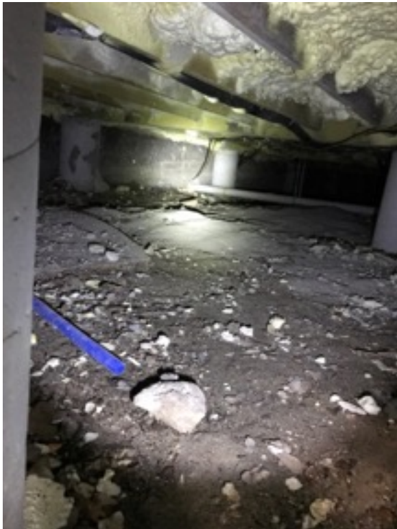
RIGHT SIDE CRAWL SPACE
